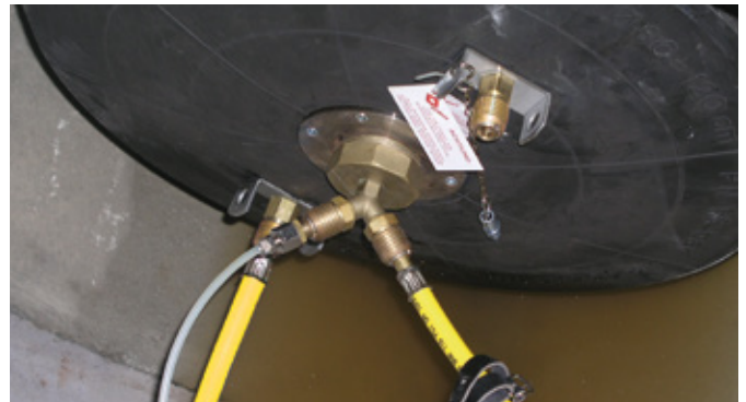
Air pressure test
